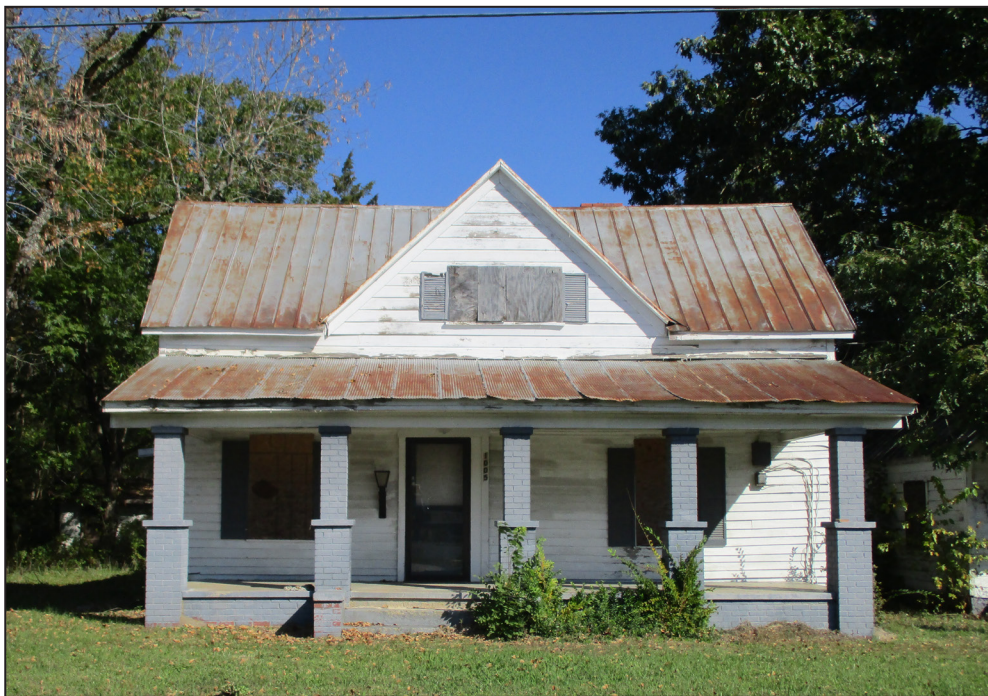
Photograph 1: Facade (south elevation) of 1005 E. 11th St.; looking north. (2016)
