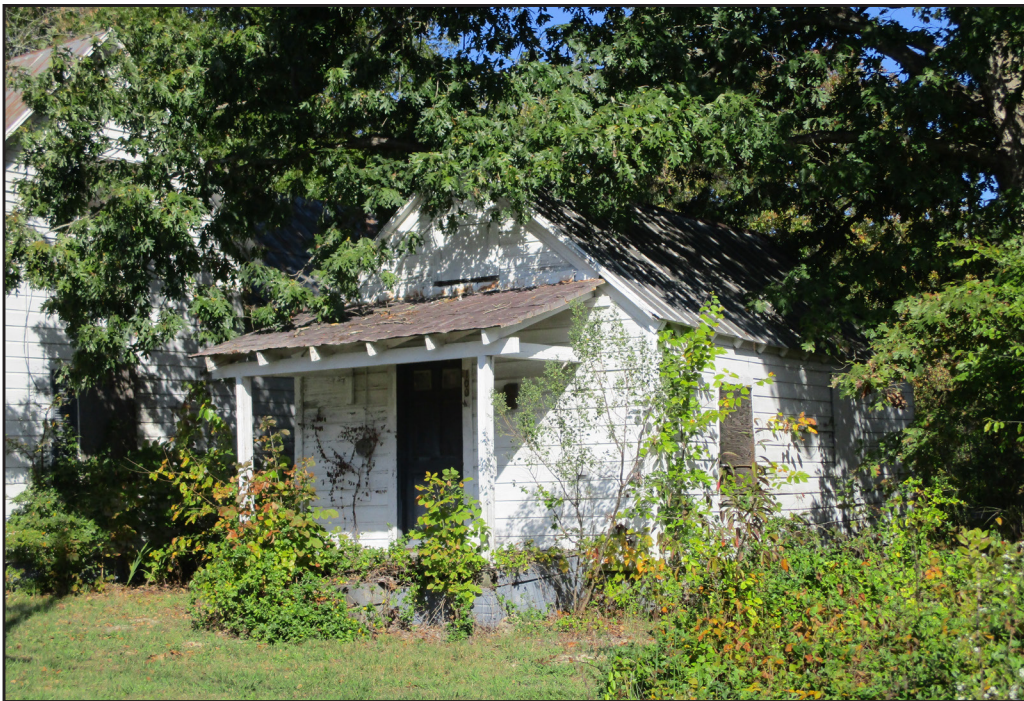
Photograph 7: Southeast elevation of 1007; looking northwest. (2016)
