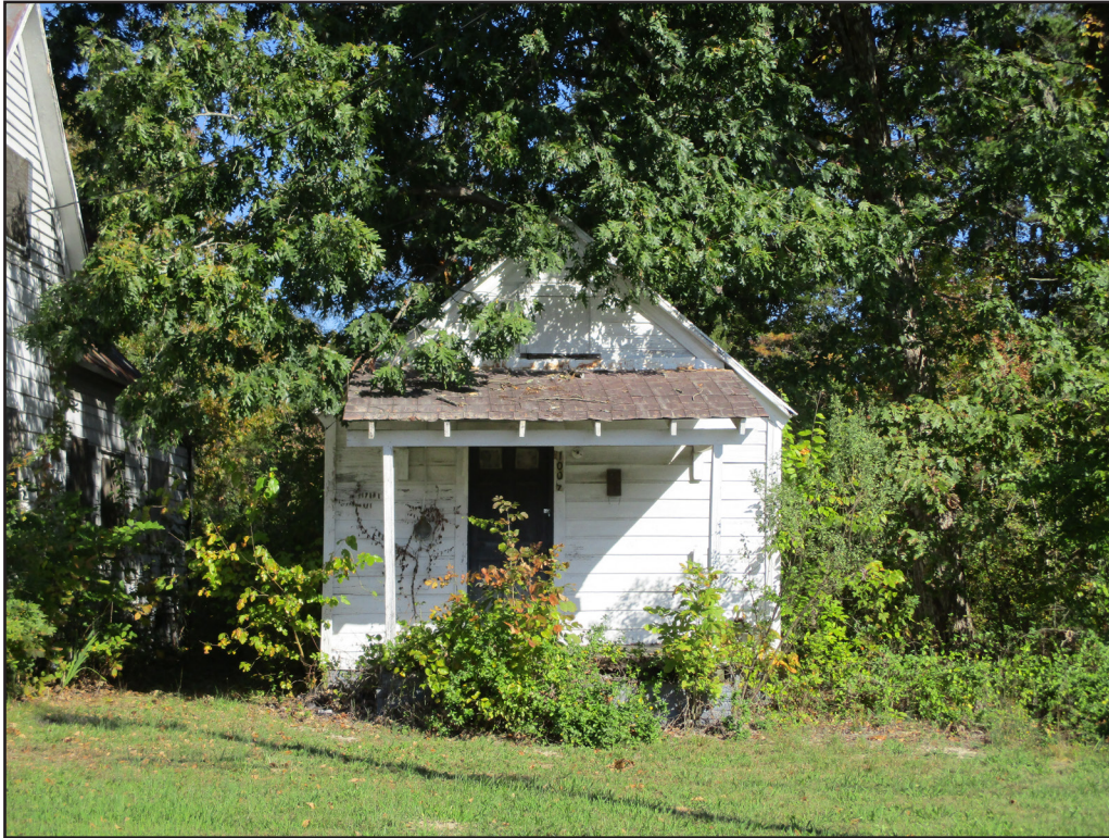
Photograph 6: South elevation of 1007 E. 11th St.; looking north. (2016)
