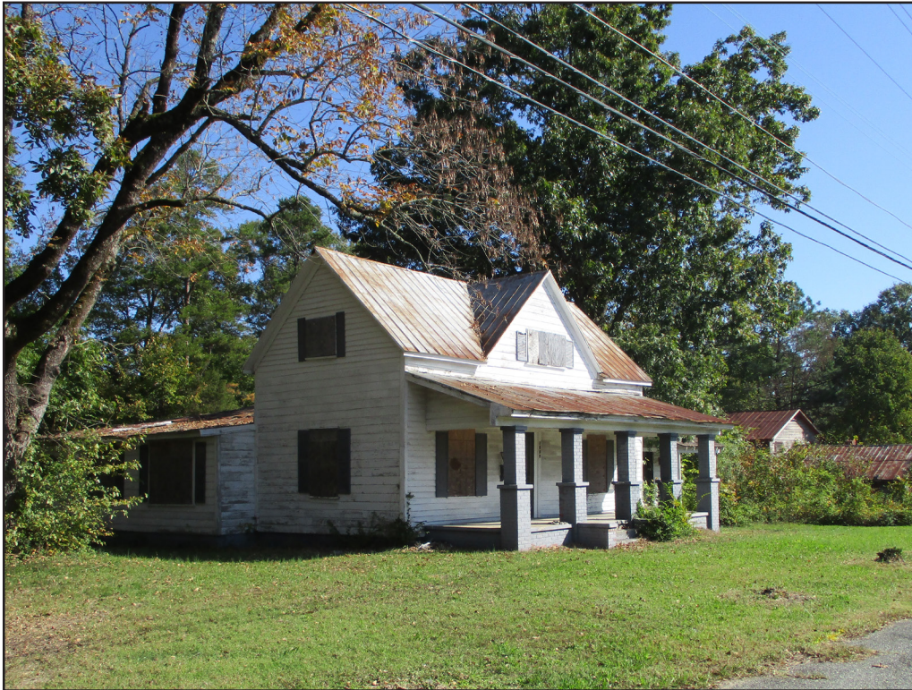
Photograph 2: Southwest elevation of 1005 E. 11th St.; looking northeast. (2016)
