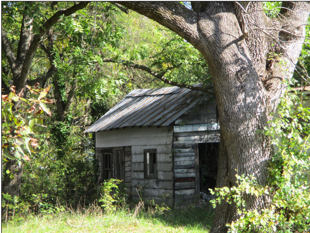
Photograph 8: Southwest elevation of rear shed. (2016)
